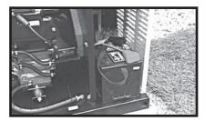
Before purchasing a battery for the generator, refer to the Installation Guide for a list of recommended batteries. Follow all of the procedures and safety precautions in the Installation Guide when installing the battery.
